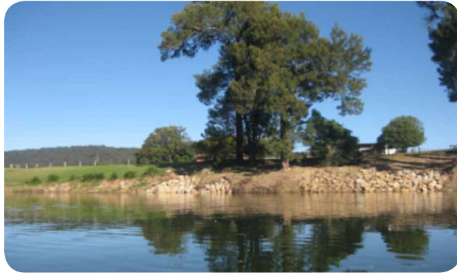
Rock revetment, Shields' property, Fernmount.
