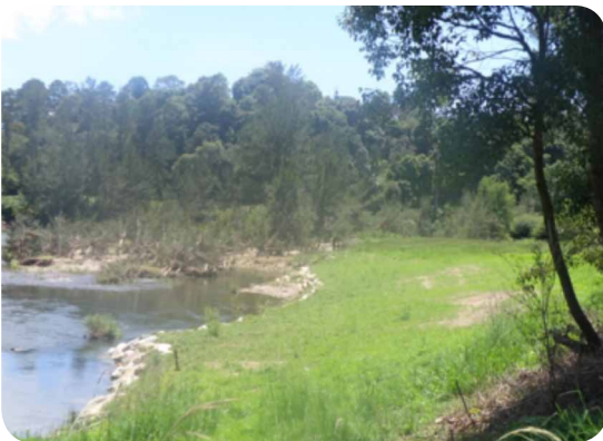
Bank battering & rock revetment, Sanger's property, Bellingin.
