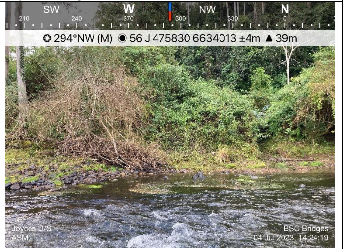
Joyces Bridge Downstream
