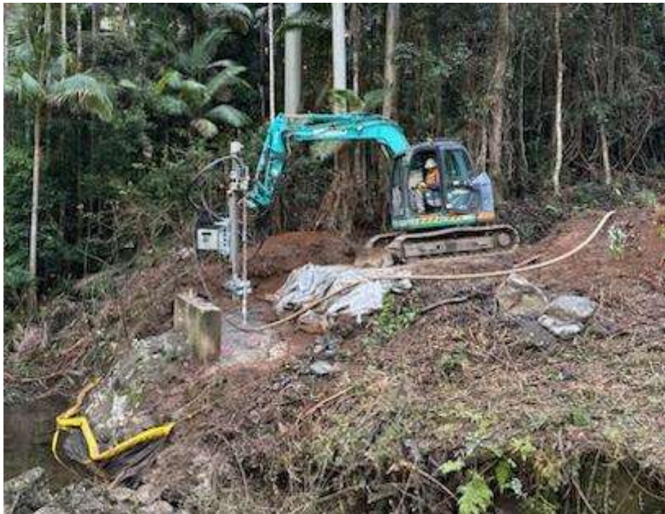
Same smaller excavator (7t) rock anchor rig
