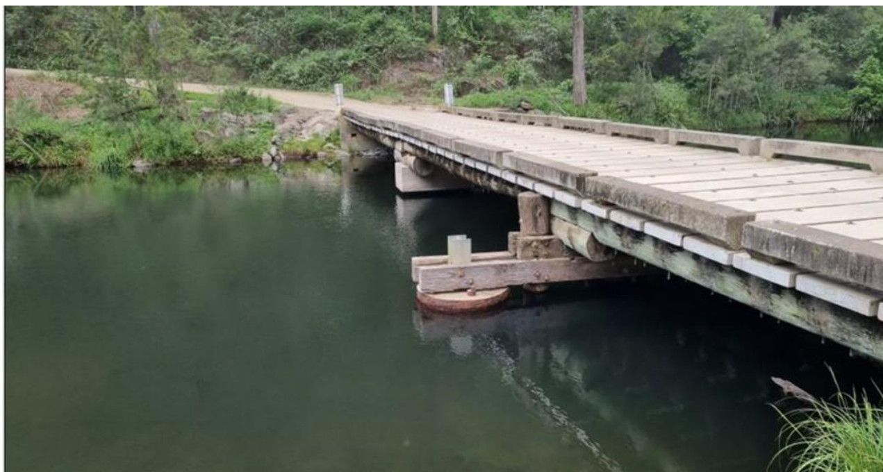
Plate 3-3 Justins Bridge – existing timber structure
