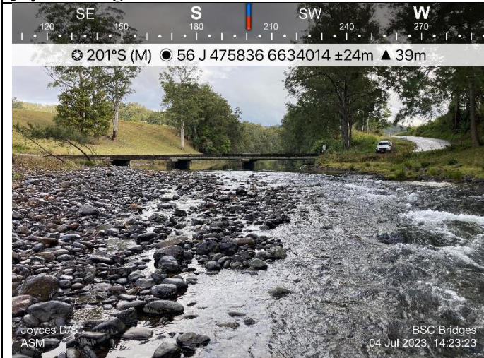
Joyces Bridge Downstream
