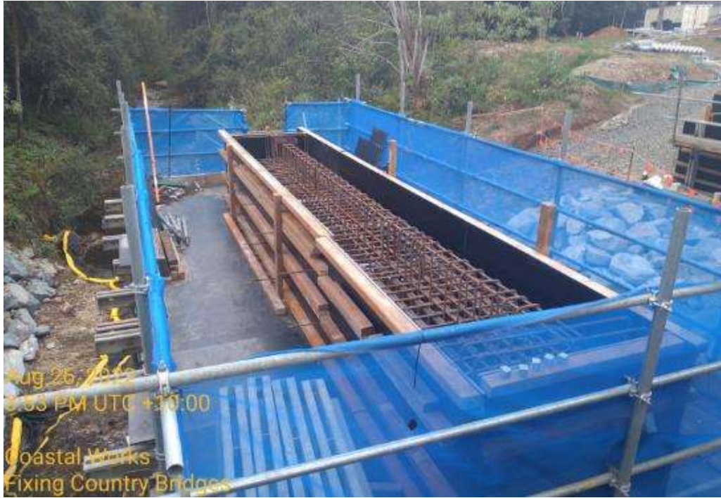
Cast in-situ headstock with elevated temporary works walkway around
