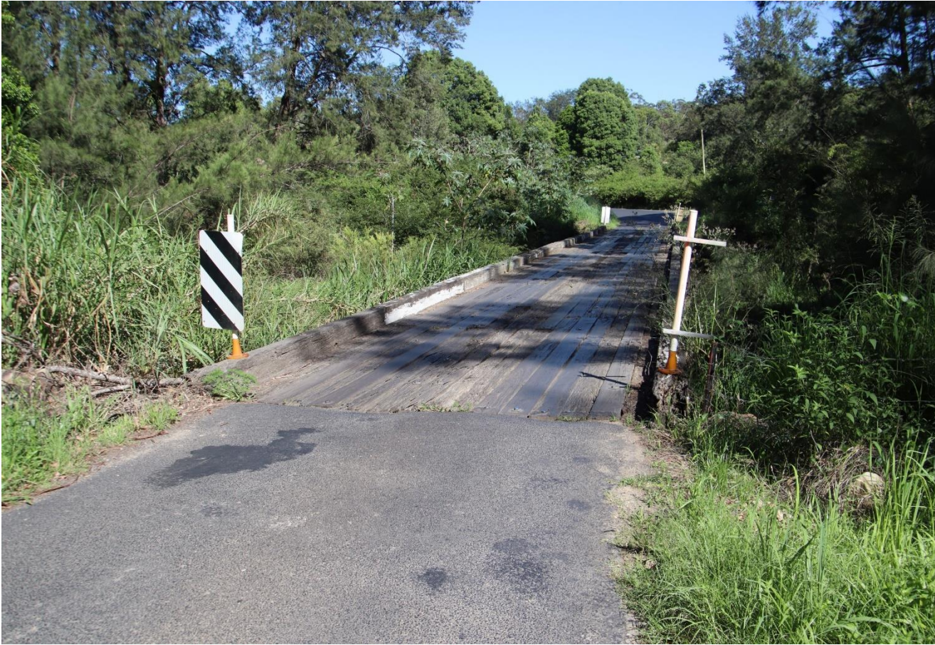
Plate 3-4 Duffys Bridge – existing timber structure
