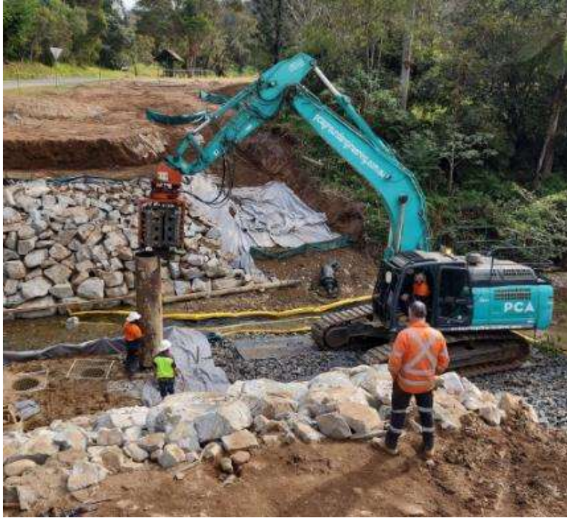
Excavator with 2t vibratory unit used to pitch steel pile liners
