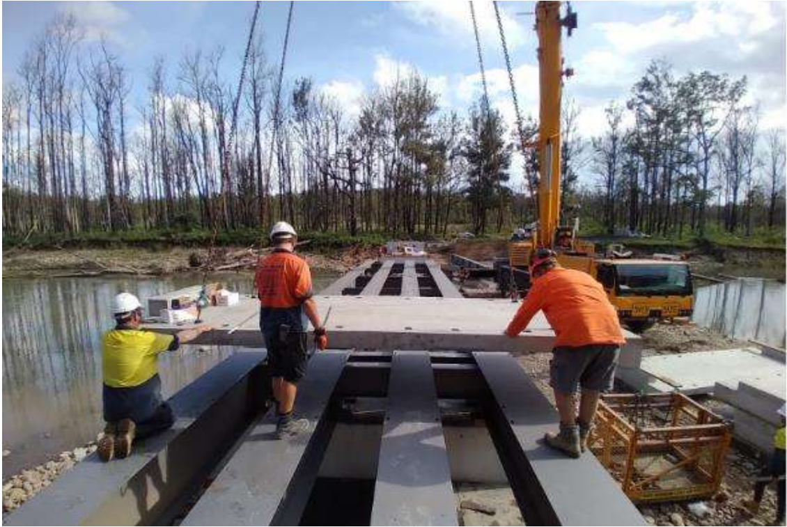
Landing precast concrete panels onto steel girder span
