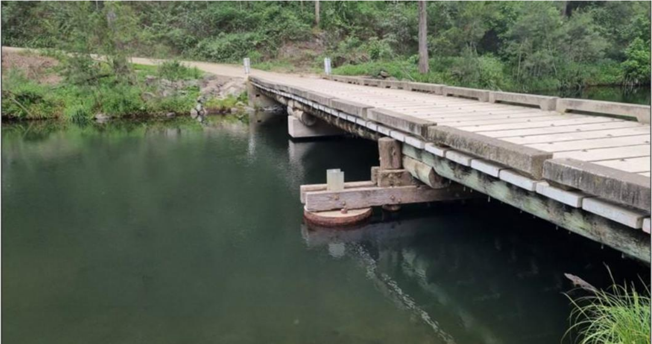
Plate 1.3 Justins Bridge – existing timber structure
