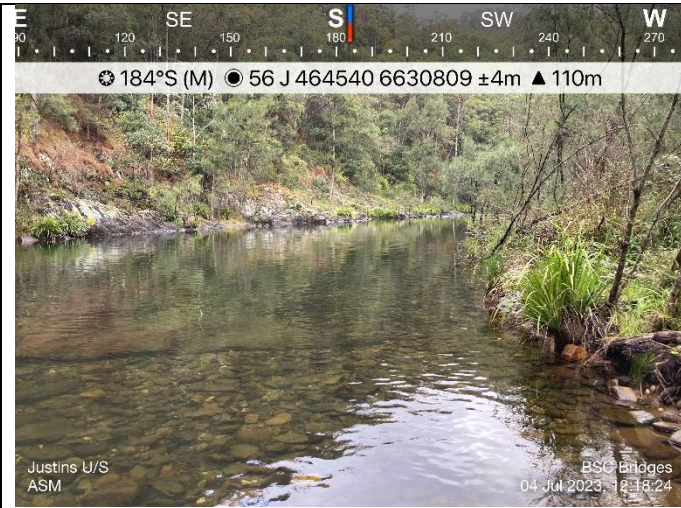
Justin's Bridge Upstream
