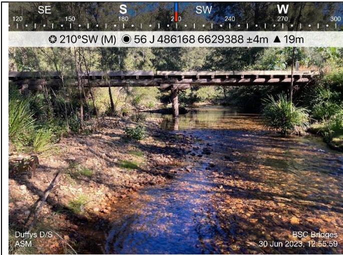
Duffys Bridge Downstream
