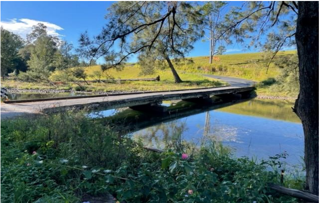
Plate 1.1 Joyces Bridge – existing timber structure
