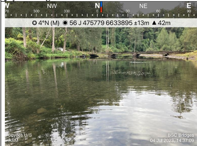
Joyces Bridge Upstream
