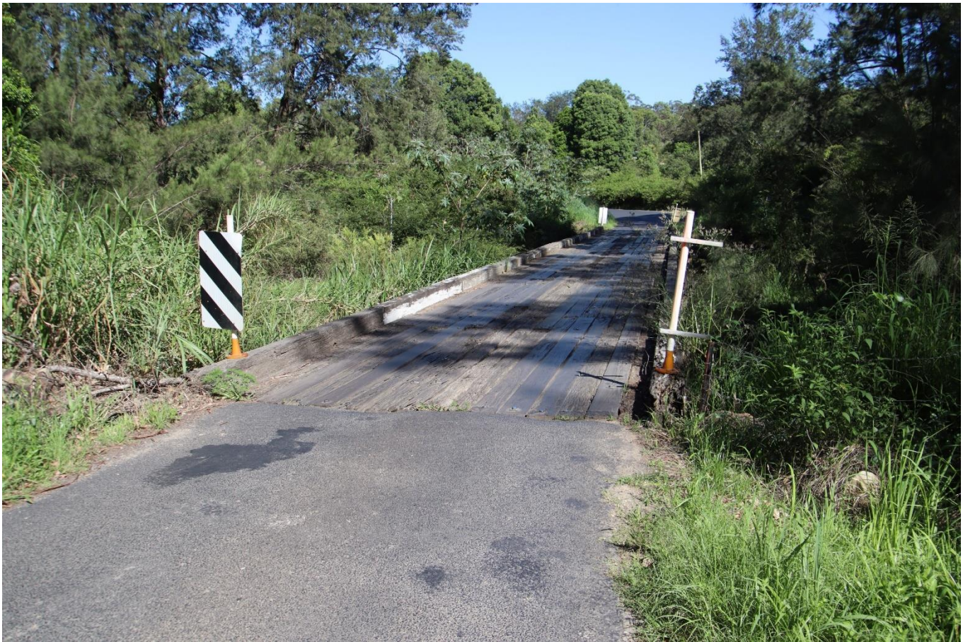
Plate 1.4 Duffys Bridge – existing timber structure
