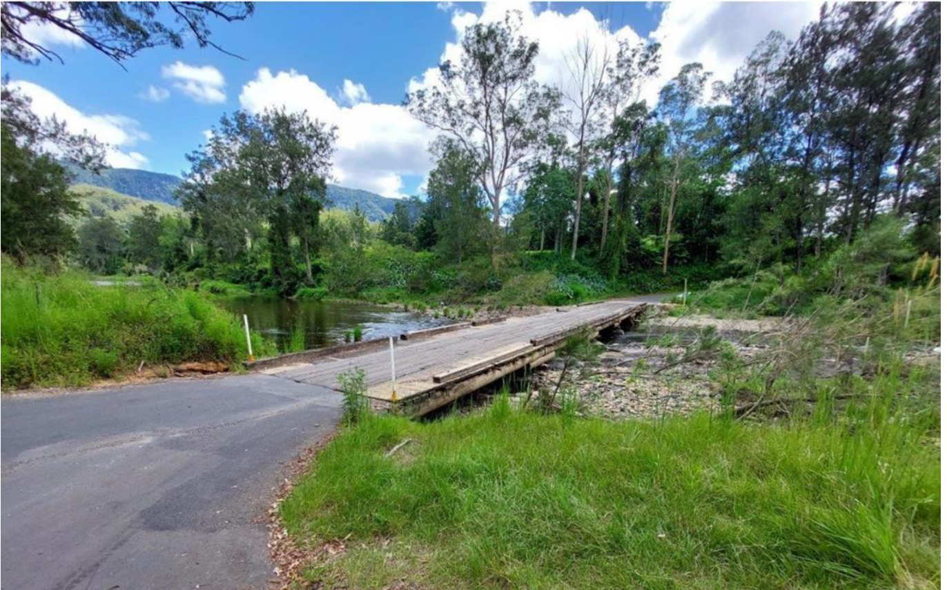
Plate 1.2 Hobarts bridge – existing timber structure
