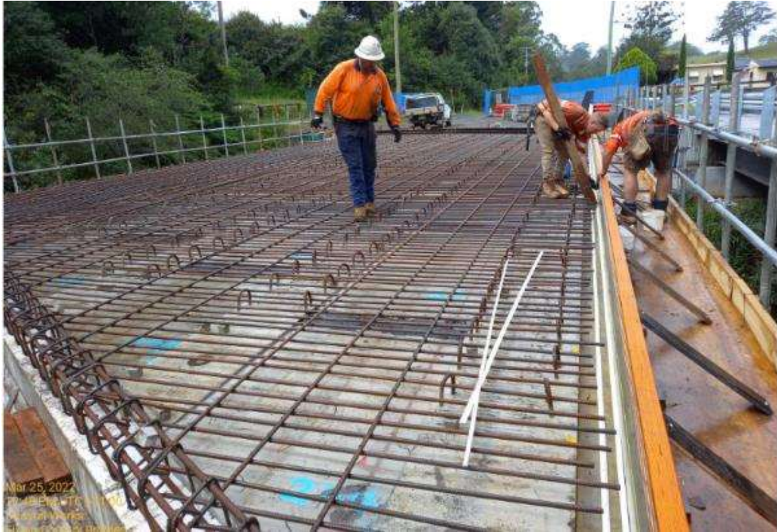
Concrete deck pour with elevated walkway attached to bridge planks
