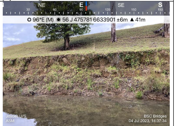
Joyces Bridge Upstream
