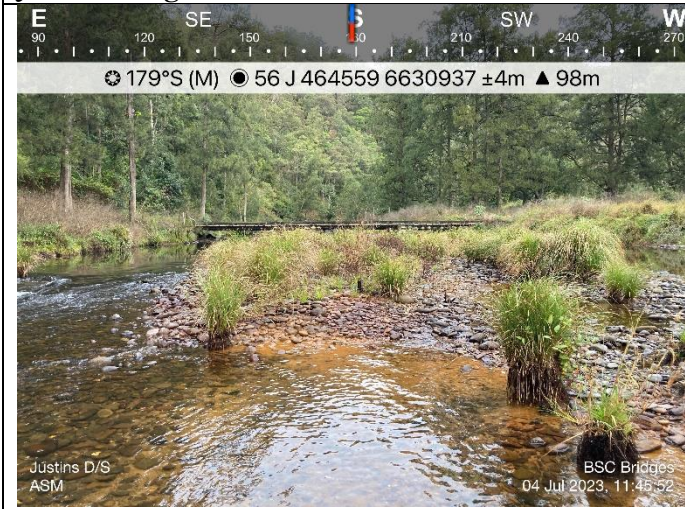
Justins Bridge Downstream
